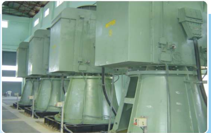
INDI Lift Irrigation Scheme Vertical Mixed Flow Pump 17892 Cum/hr x 35 m x 2.1 MW
