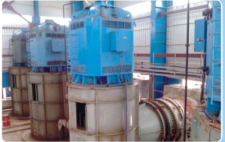
CW Pump for NTPC Aravali Power- Indira Gandhi STPP (3x500MW) Vertical Mixed Flow Pump - 30000 Cum/hr x 27 m x 2.8 MW
